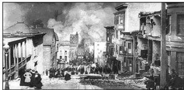
Fig 1.3: San Francisco burning after the 1906 Earthquake
