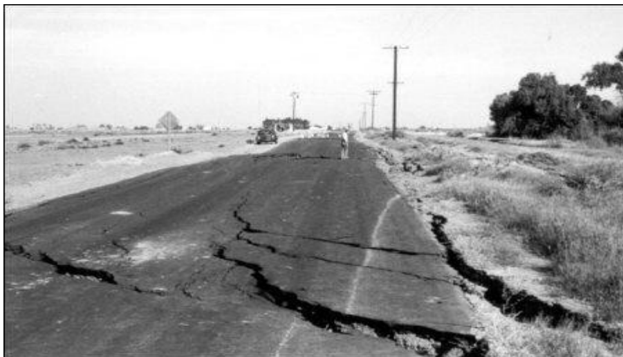
Fig 1.2: Ground displacement
