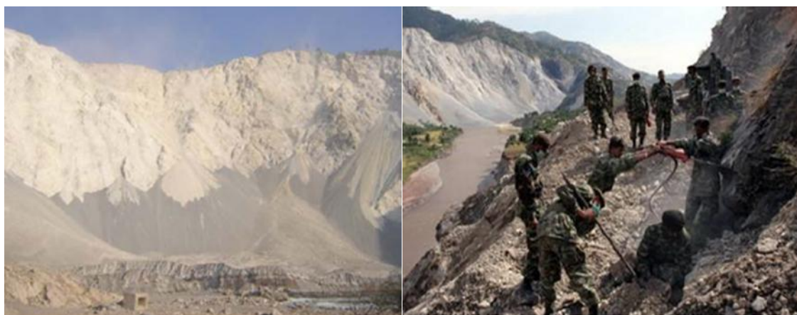
Fig 1.4: Slope failure observed in the regions of Balakot and Muzaffarabad (Pakistan Earthquake 8 th Oct. 2005.)
