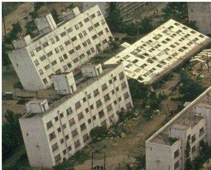
Fig 15.1: Apartment buildings tilted by liquefaction-induced loss of bearing strength during the 1964 Niigata, Japan, earthquake.
