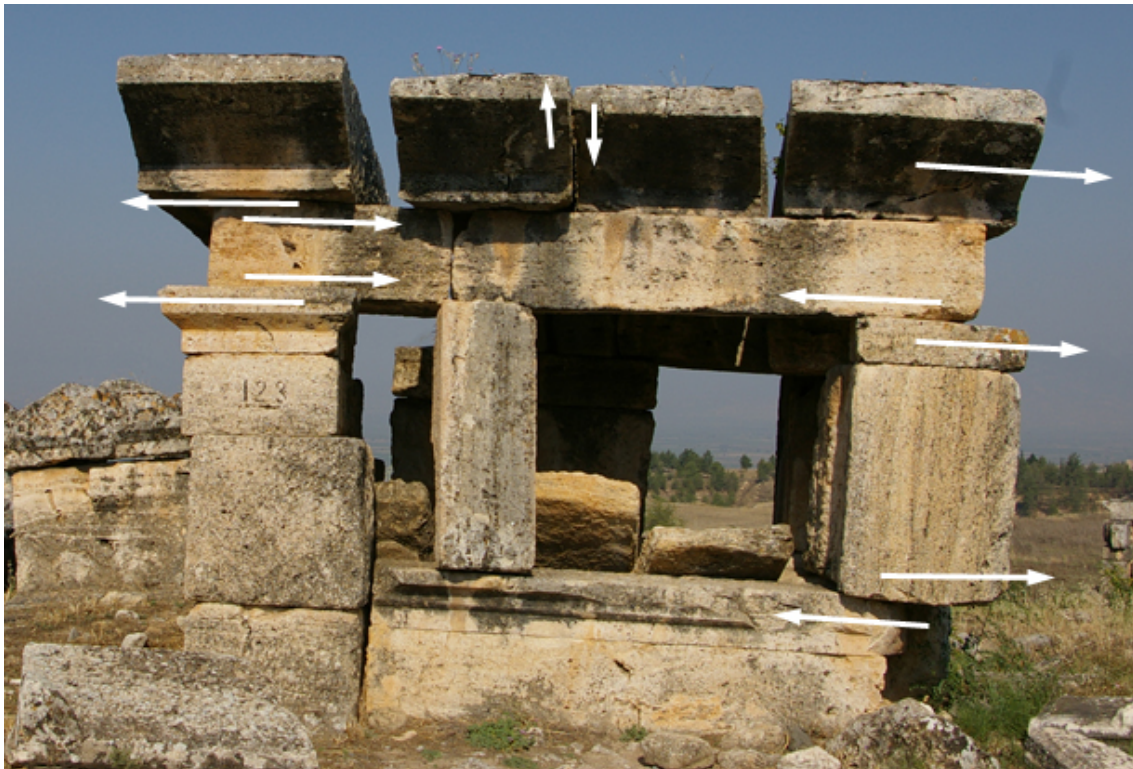
Fig. 2.13 - Ruins of a tomb in Hierapolis, an ancient city in Turkey founded around 200 B.C. and abandoned after an earthquake in 1534. Many offsets can be observed between the different blocks: although gravity may be a primary driver of this tomb deformation, perhaps occasional seismic shakings contributed (taken from Callan Bentley in AGU Blogosphere).
