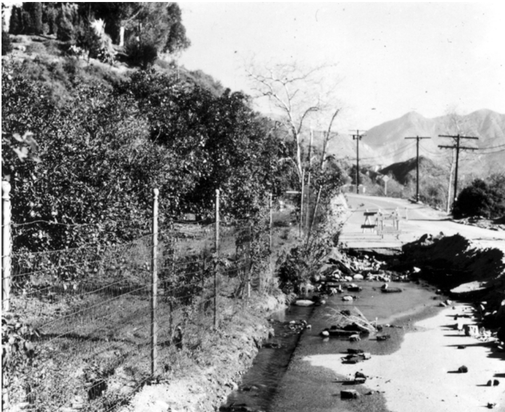
Fig. 1.72 - San Fernando earthquake of February 9, 1971. Trace of the main reverse fault where it crosses Little Tujunga Road. By the time this photograph was taken a dirt ramp at right had been built up the scarp. The scarp indicates more than 1-m reverse dip-slip movement. The fence indicates little strike-slip displacement at this place, which is near the last end of the line of surface rupture.
