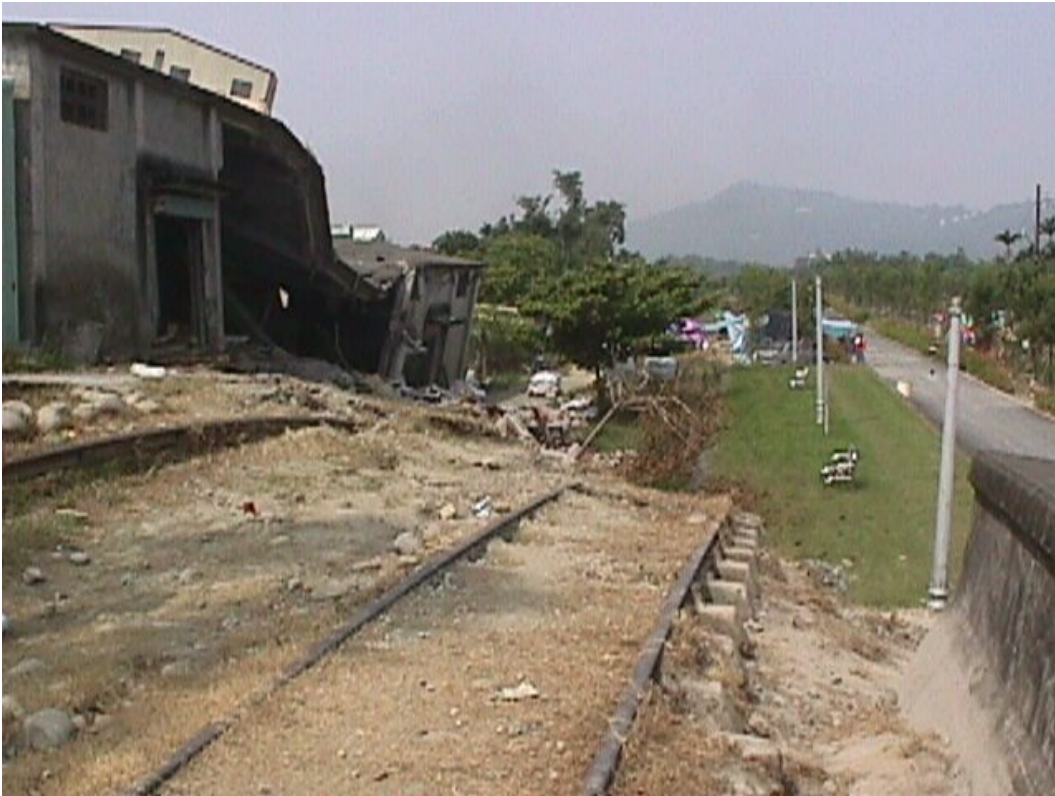
Fig. 1.81 - Chichi (Taiwan) earthquake of 1999. Behind the building complex (upper left), the fault offset the originally level ground and railroad tracks by about 3 m vertically.
