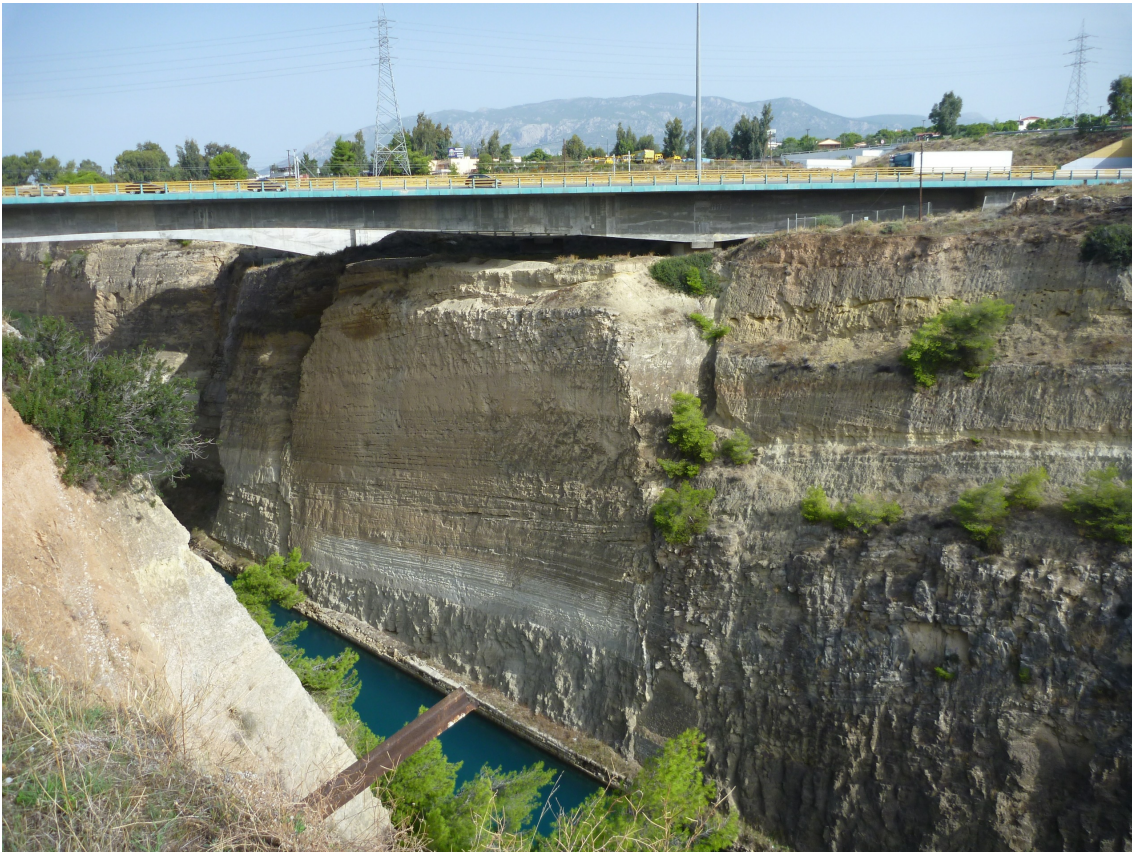
Fig. 2.12 - Trace of a fault in the Gulf of Corinth that was activated during several ancient earthquakes and also during the 1981 seismic sequence.
