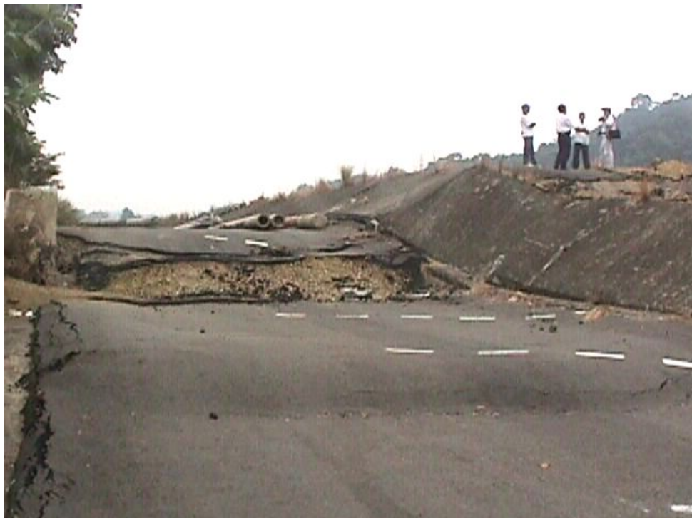
Fig. 1.80 - Chichi (Taiwan) earthquake of 1999. The fault tore up the adjacent road and levee in a narrow and relatively uncomplicated pattern.
