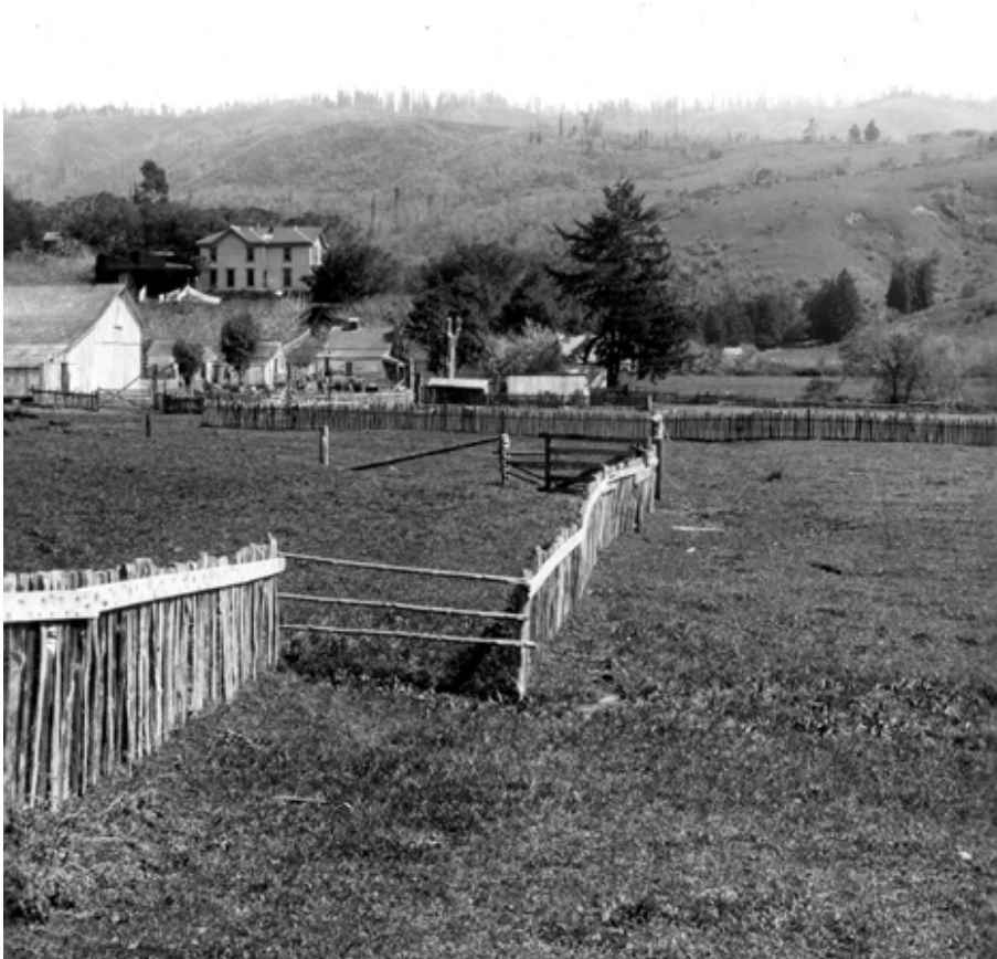
Fig. 1.68 - Fence offset by the causative fault of the San Francisco earthquake of April 18, 1906, on ranch of E.R. Strain, 1 1/2 miles north of Bolinas Lagoon, looking NE. The sheer offset is 8 1/2 feet; the total displacement, shown partly by crooking of fence, is 11 feet (from the USGS website).
