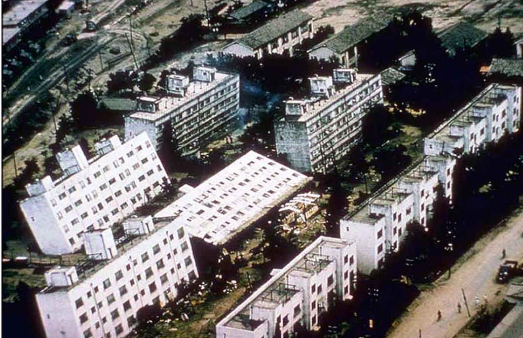
Fig. 1.48 – Effects of liquefaction during the 1964 Niigata earthquake.
